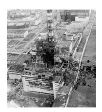
▲ In 1986, the reactor core at Chernobyl (in what is now Ukraine) overheated, exploded, and destroyed part of the containment structure. The release of radioactive nuclides into the environment forced the government to relocate over 335,000 people.
